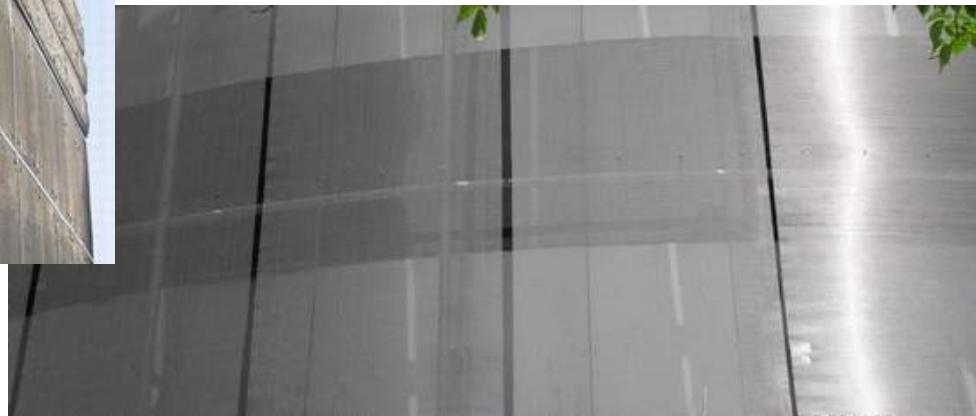
It is efficient and economy for installation. Usually, the dimensions of weave mesh are tailor-made and cut-to-size to fit the design and the installation structure. Also, it may come with fixing accessories per your design to withstand the required loads.
